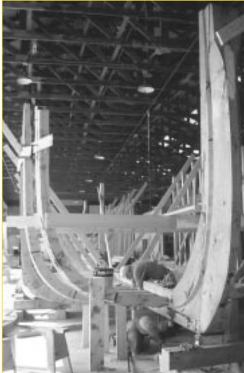
With the stem in place, cant frames are shaped and installed.
